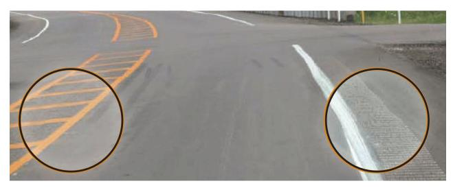
Figure 6: Lane Narrowing Using Rumble Strips
