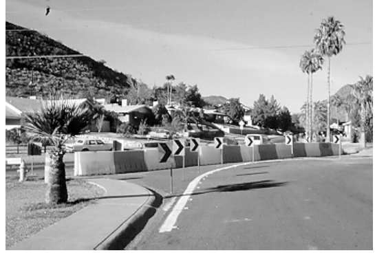
Figure 5.16. Diagonal Diverter. (6th Ave.—Phoenix, AZ)
