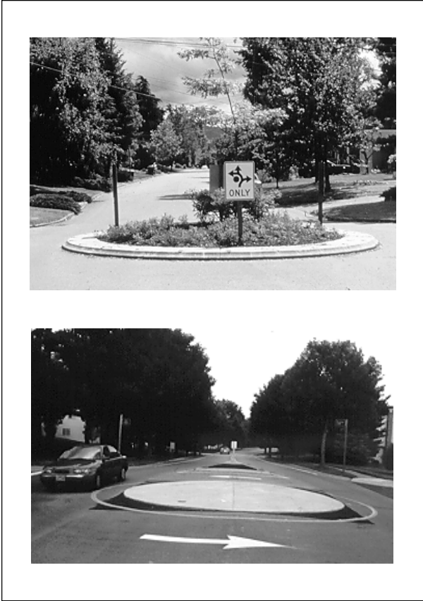
Figure 3.18. Mountable Traffic Circles. (Bellevue, WA, and Howard County, MD)
