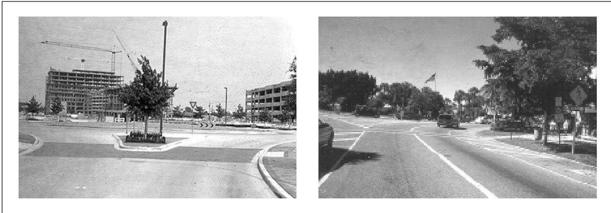
Figure 3.23. Modern Roundabout (left) versus Old-Fashioned Traffic Circle (right). (Dallas, TX, and Sarasota, FL)
