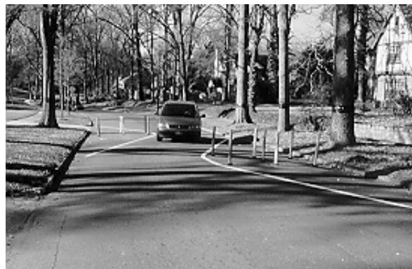
Figure 4.19. Temporary One-Lane Chicane. (Charlotte, NC)
