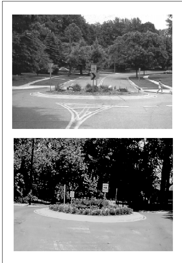
Figure 4.30. Traffic Circles in the Same Jurisdiction Signed and Marked Differently. (Montgomery County, MD)
