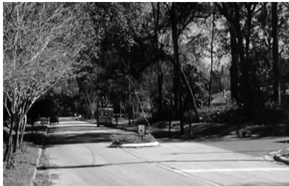
Figure 6.1. Ineffective Traffic Circle at a T-Intersection. (Gainesville, FL)
