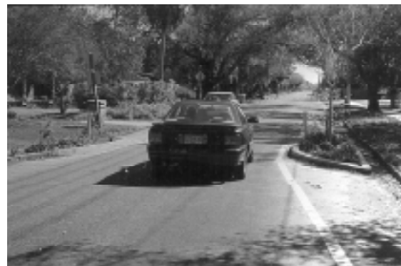
Figure 3.34. Unsuccessful One and One-Half Lane Choker. (Sarasota, FL)
