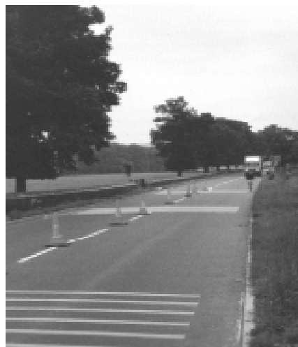
Figure 9.7. “Jiggle Bars” on an Approach to Town.
