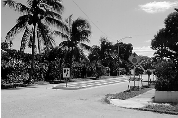
Figure 3.32. Center Island Discouraging High-Speed Turns. (West Palm Beach, FL)
