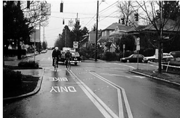
Figure 7.12. Half Closure that Discourages Violations. (Portland, OR)
