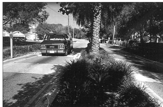
Figure 3.38. Speed Table Combined with a Center Island Narrowing. (Sarasota, FL)
