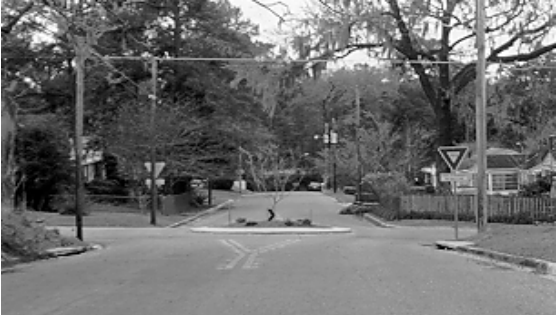
Figure 3.17. Blocking the Straight-Through Movement. (Tallahassee, FL)
