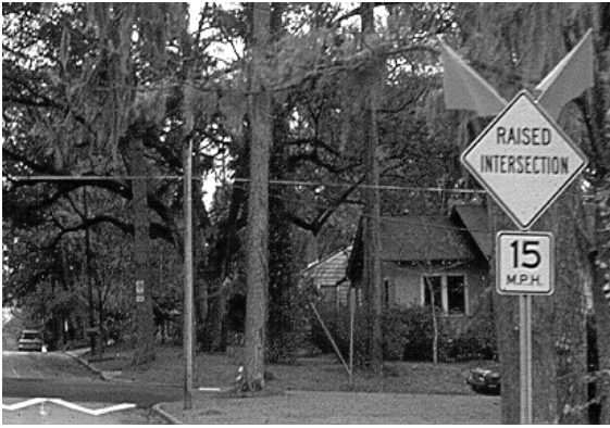
Raised Intersection. (Tallahassee, FL)
