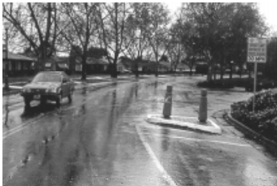
Figure 5.40. Photo-Radar Warning Sign Combined with a Choker. (San Jose, CA)
