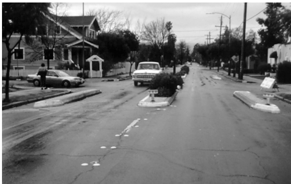
Figure 6.7. Tight Geometrics at the Site of a Bicycle Accident. (San Jose, CA)
