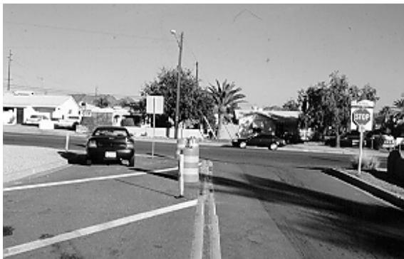
Figure 7.11. Half Closure that Invites Violations. (Phoenix, AZ)
