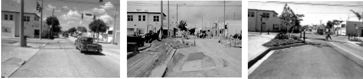
Figure 1.8. Before, During, and After Commercial Area Revitalization. (West Palm Beach, FL)
