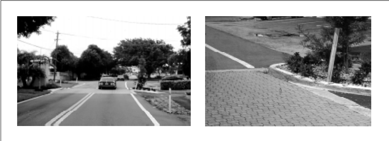
Figure 6.13. Problem Choker After Improvement. (Ft. Lauderdale, FL)
