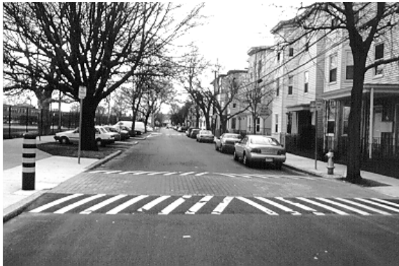
Figure 5.8. Raised Crosswalks/Raised Intersection/Chicane. (Berkshire St.—Cambridge, MA)
