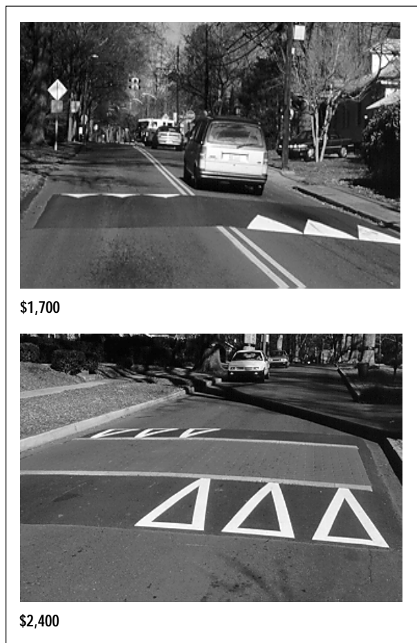
Figure 3.14. Plain (above) and Stamped (below) Asphalt Tables with Cost Estimates. (Charlotte, NC)
