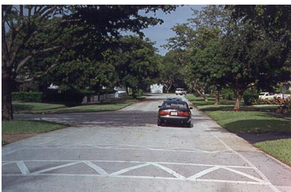
22-foot Hump. (Ft. Lauderdale, FL)
