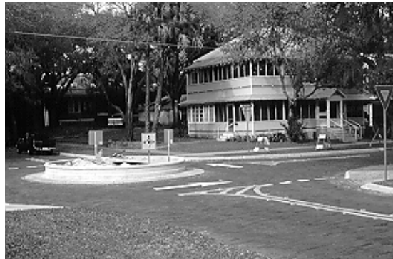
Figure 7.13. Traffic Circle with a 2-inch Lip to Accommodate Fire Trucks. (Orlando, FL)
