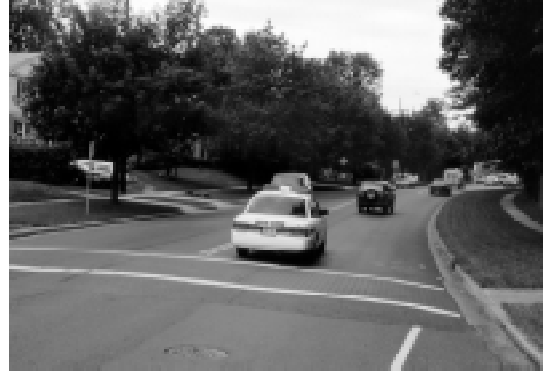
Figure 5.10. 22-foot Raised Crosswalks. (Bel Pre Rd.—Montgomery County, MD)
