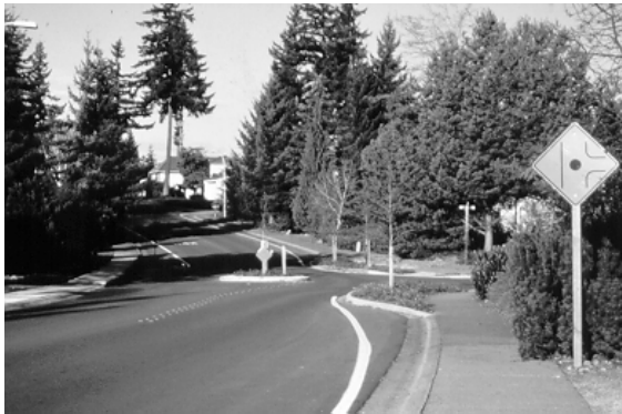
Figure 3.35. Traffic Circle Combined with Neckdowns. (Bellevue, WA)
