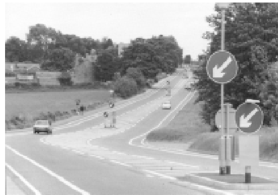
Figure 9.3. Reallocation of Right-of-Way without Deflection.
