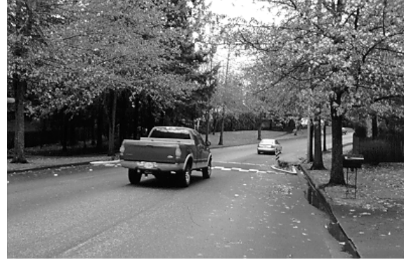
Figure 9.11. Speed Table with Curb Extensions on a Neighborhood Collector. (Beaverton, OR)
