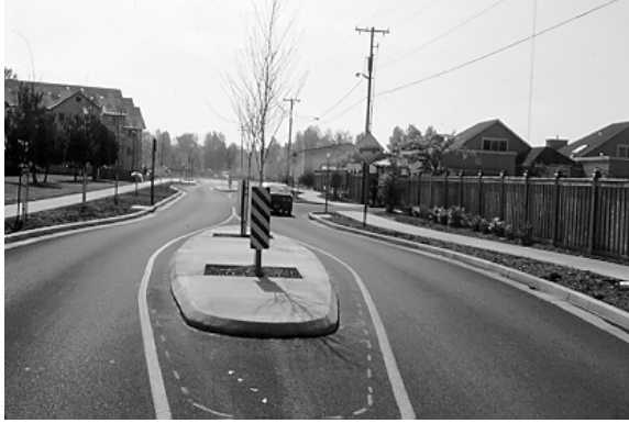
Figure 7.18. Scaled Down Deflector Island with Reduced Effectiveness. (Eugene, OR)
