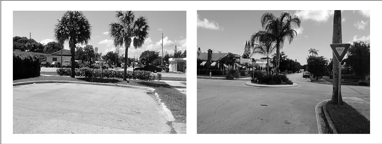
Figure 3.4. Early Closure and Later Traffic Circle. (West Palm Beach, FL)
