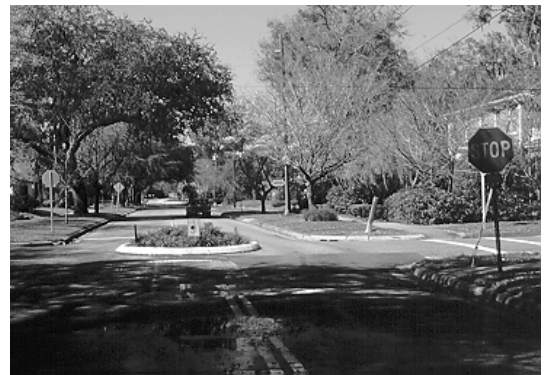
Figure 5.12. 10-foot Diameter Traffic Circle. (NE 10th Ave.—Gainesville, FL)
