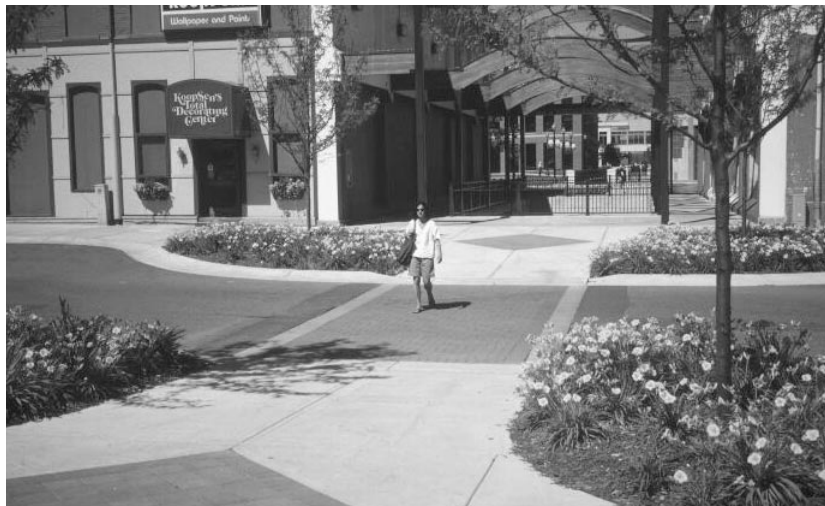
This midblock crossing is in Kalamazoo, Michigan. The landscaping and textured crosswalk are visually appealing and provide a clear message about where pedestrians can be expected to cross the street.
