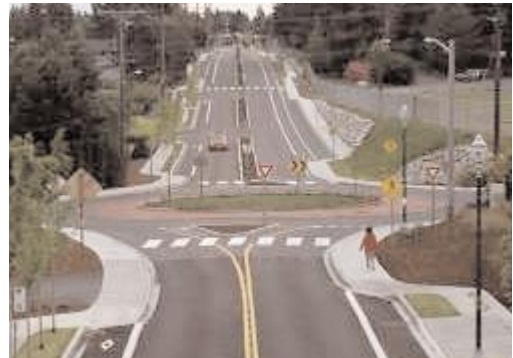
The addition of bicycle lanes and sidewalks created space for pedestrians while medians and landscaping narrow the street width and slow traffic.
