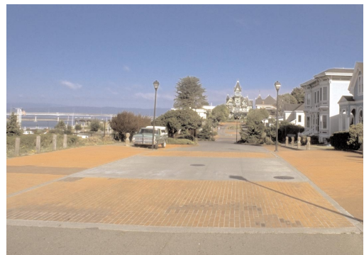
Part of Eureka's Second Street streetscaping featuring a raised intersection, brick crosswalks and Carter Mansion in the background.
