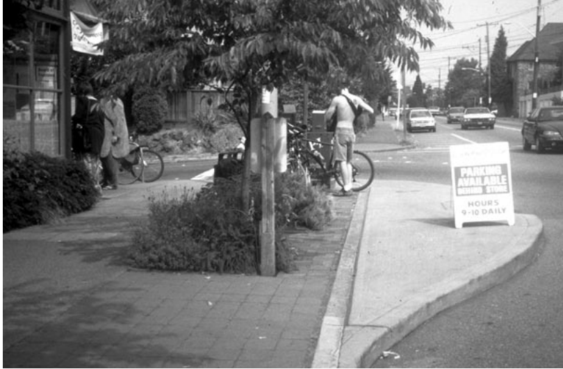
A curb extension on an arterial street in Seattle, Washington. The crossing distance for pedestrians is substantially reduced by the installation of this device.
