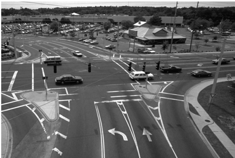
Well designed slip lanes at a busy, wide intersection. The crosswalks are located to allow the greatest visibility between the drivers and pedestrians.
