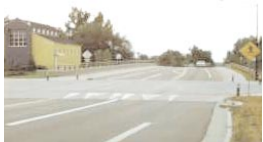
A raised intersection, designed to reduce traffic speeds and facilitate pedestrian crossings.
