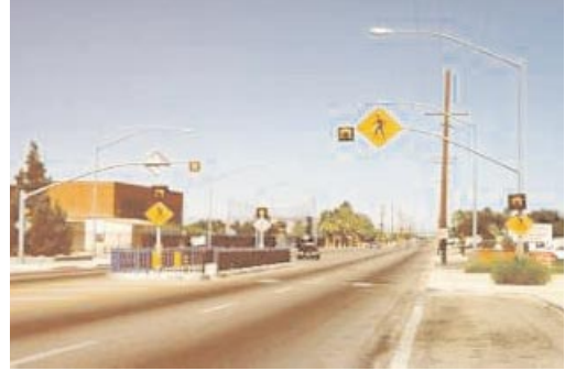
The gates on this pedestrian island direct students' attention to the oncoming traffic.
