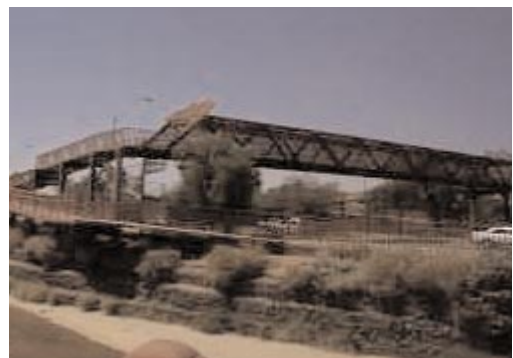
A recycled bridge provides a safe pedestrian route for students in Phoenix
