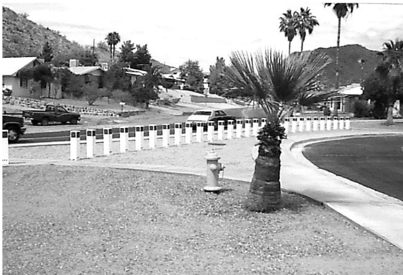
Access is closed on this residential street in Phoenix, AZ.
