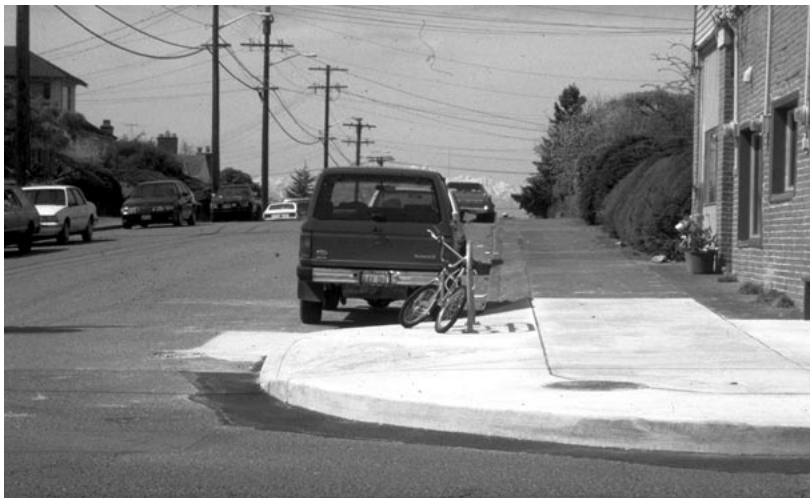
A curb extension on a residential street, also in Seattle, Washington. In addition to improving pedestrian safety at this intersection, the bulb provides additional sidewalk space for a bicycle rack.
