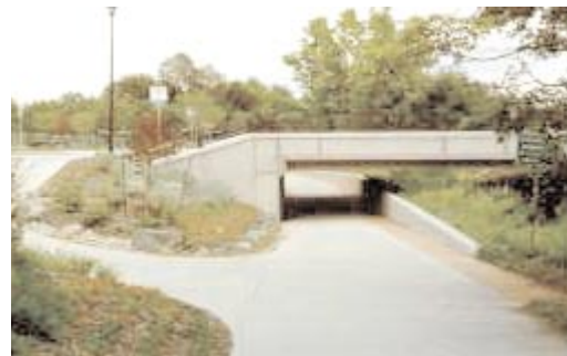
A pedestrian underpass which filled a gap in Boulder's existing trail system.
