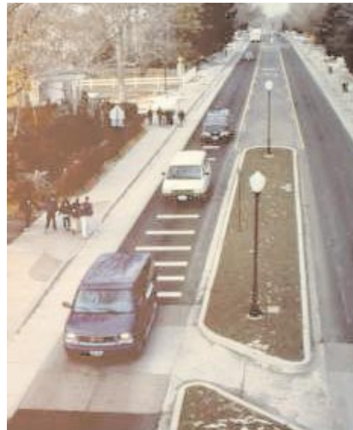
Wider sidewalks, bike lanes and raised crosswalks with a crossing island create a safer environment.
