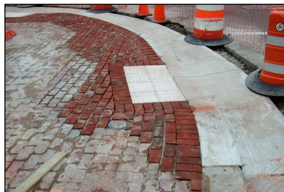
Image 7: Bricks and pavers that have come loose or are not evenly placed can create a hazard.
