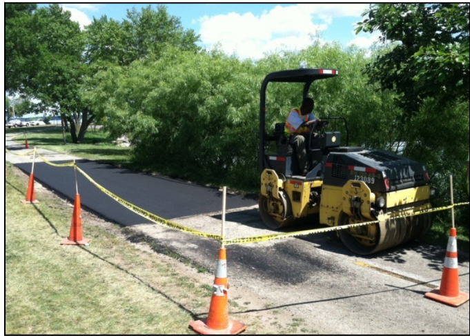
Image 6: Section of a shared use path being repaired in Madison, Wisconsin
