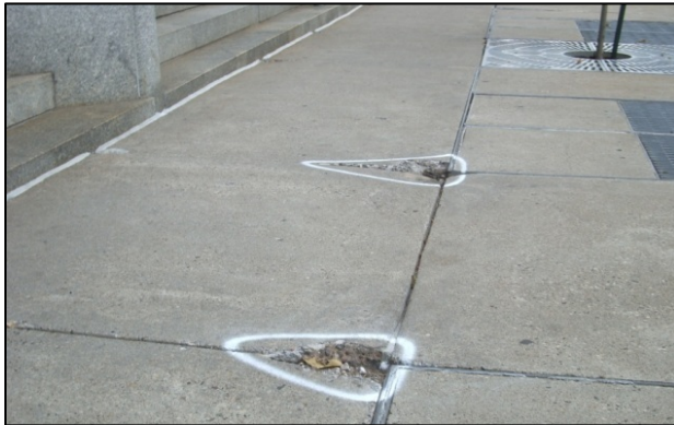
Image 10: Missing areas of concrete have been marked for repair.
