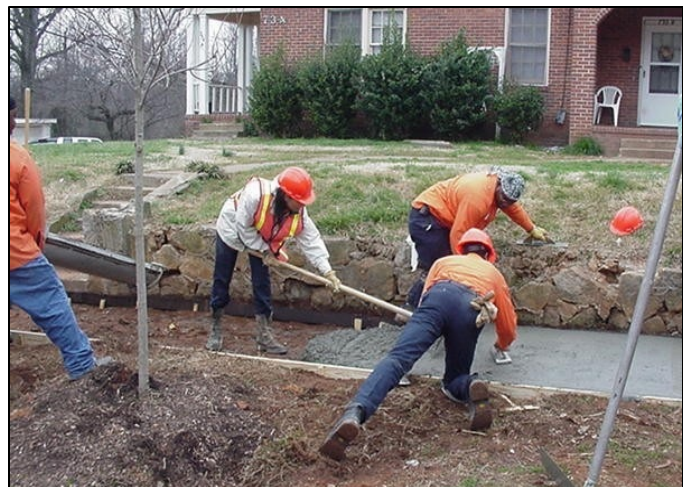
Image 16: Replacement sidewalk being installed. Photo Courtesy of the City of Charlotte
