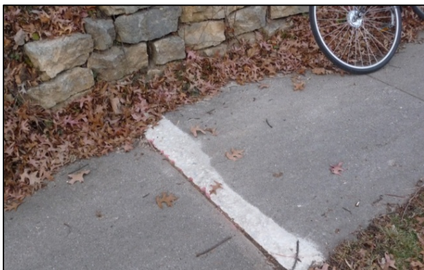
Image 12: A raised sidewalk block has been ground down to provide a smoother transition.
