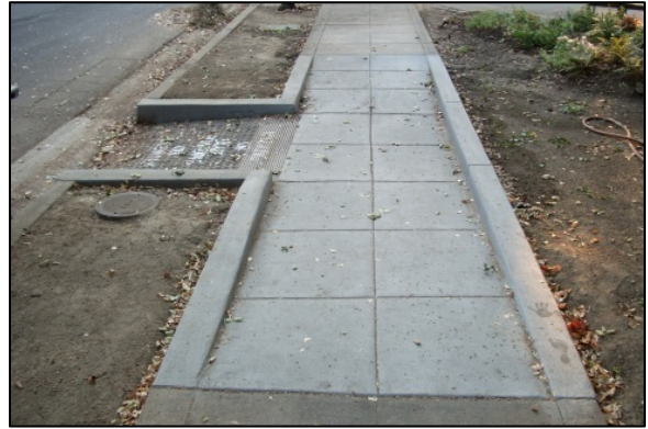
Image 1: A concrete sidewalk and curb ramp
