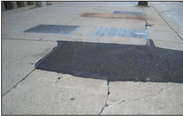
Image 8: A wedge has been placed to mitigate the hazard caused by a raised sidewalk slab.
