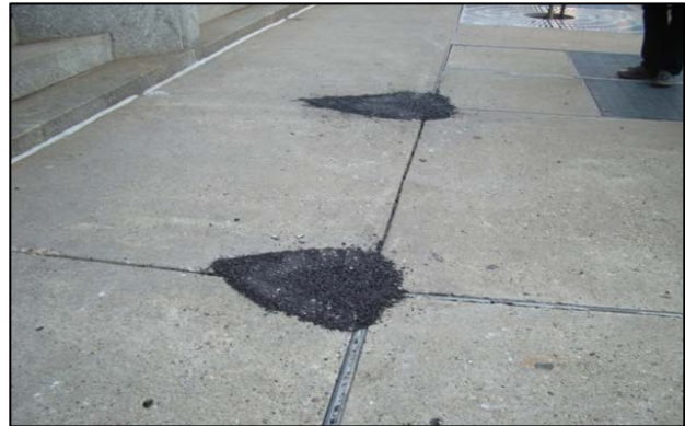
Image 11: The areas have been temporarily repaired with asphalt patches.
