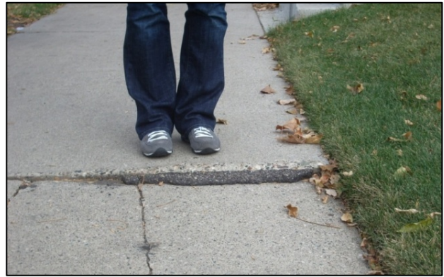
Image 9: A small wedge may still create a hazard or be difficult to navigate in a wheelchair.
