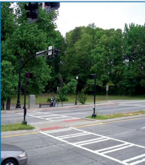
Figure 7. PHB installed on Buford Highway near pedestrian attractors: a transit stop. Photo credit: Bruce Landis
