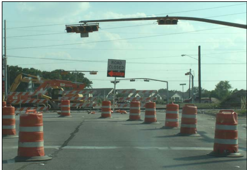
Figure X-44. Channelizing Drums Guiding Drivers through a Work Zone at an Intersection.
