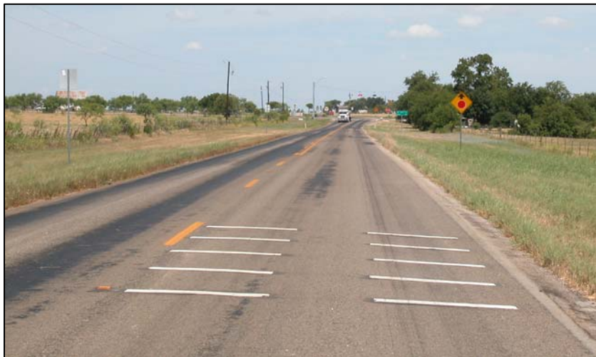
Figure X-43. Rumble Strips at Non-Work Zone Location.
