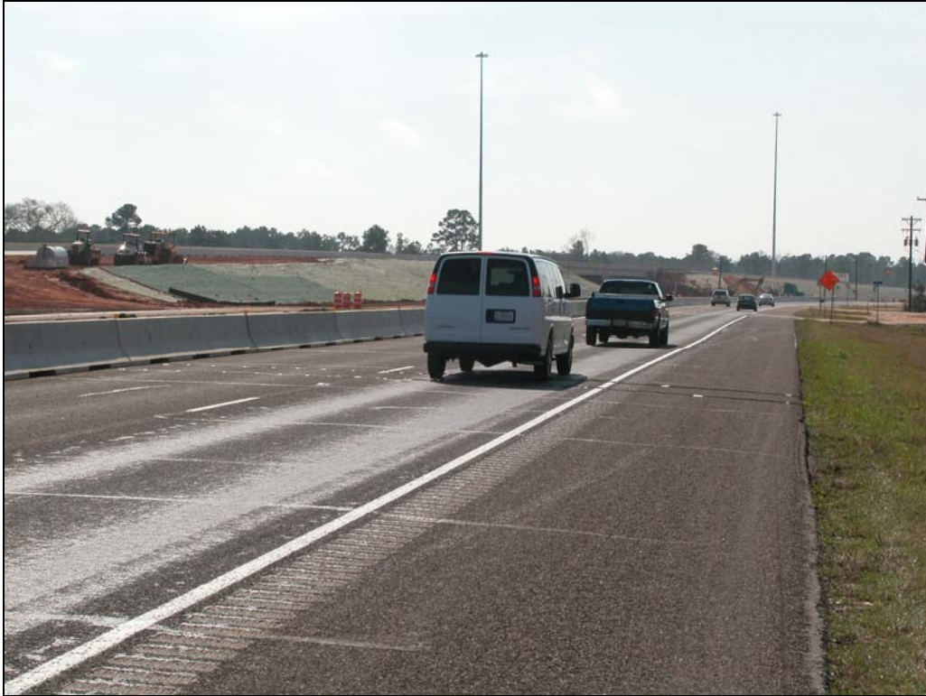
Figure X-16. Construction of Overpass Adjacent to Active Travel Lanes.
