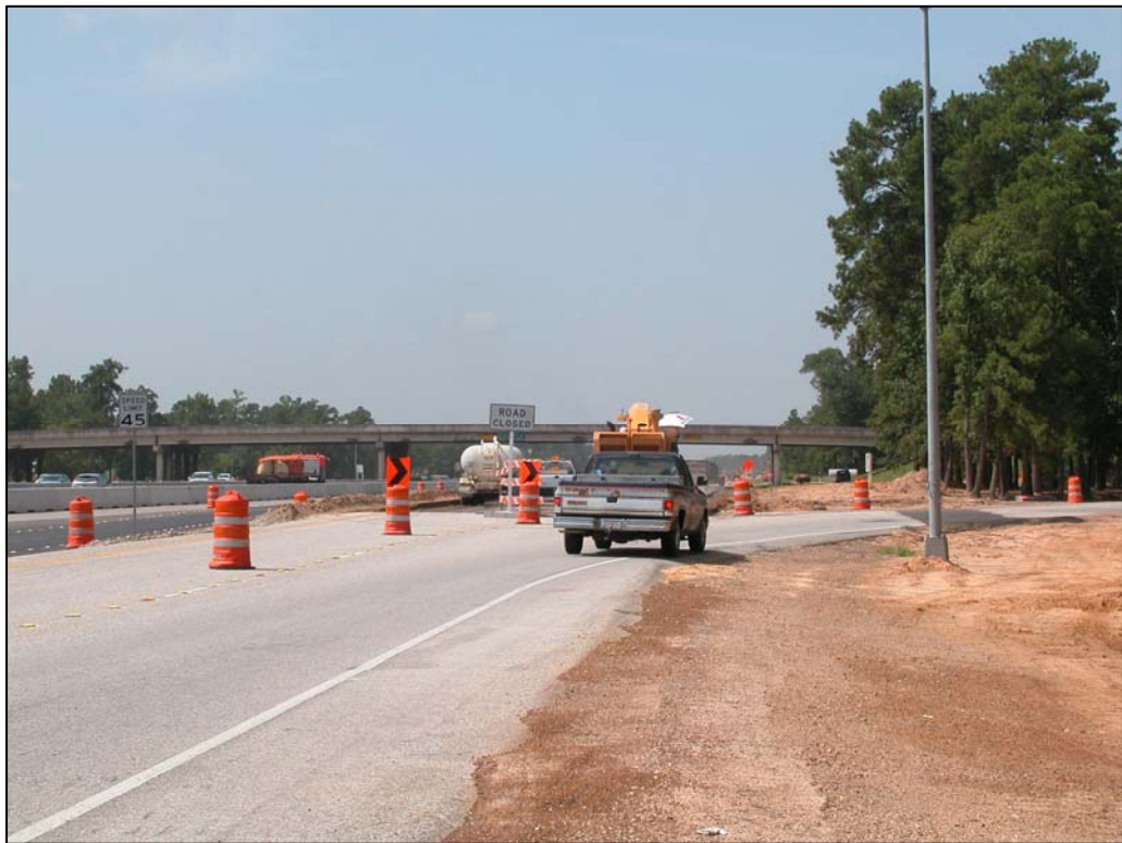
Figure X-19. Road Work in Close Proximity to Through Traffic.
