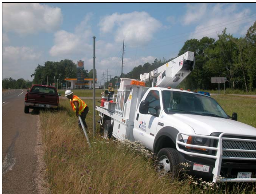
Figure X-12. Localized Maintenance (Sign Replacement).
