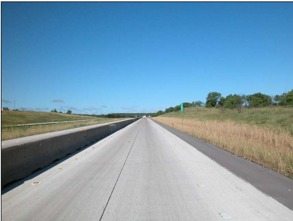
Figure X-15. Traffic Diverted to One Lane on a Reconstruction Project.
