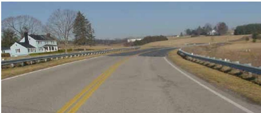
**Figure 20. Example bituminous surface treatment.**
