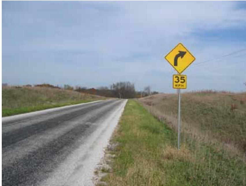
**Figure 19. Horizontal curve warning sign with speed advisory plaque.**
