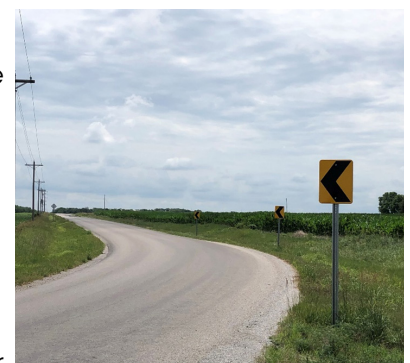
Figure 1. Chevrons at a horizontal curve in Kansas. Source: KDOT.
