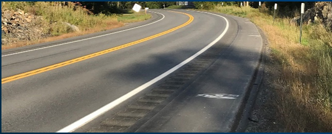
Figure 4. Center line and edge line rumble strips on a horizontal curve in Maine. Source: Maine DOT.
