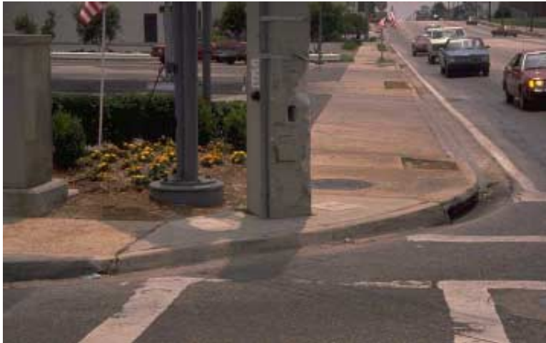
Utilities and the lack of curb cuts makes this intersection very unsafe, limits the mobility of pedestrians, and does not allow for handicapped access.
