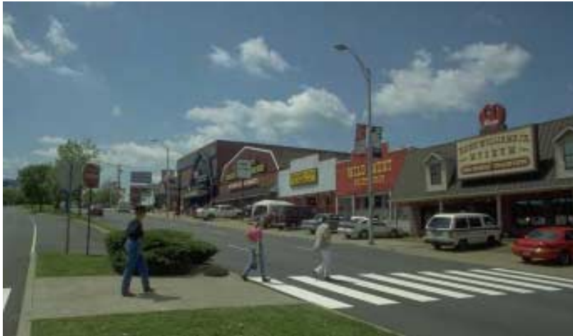
Medians and crosswalks should be placed at destination locations such as this shopping center.
