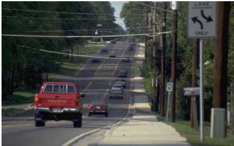
Sidewalks with a landscape strip should be installed to minimize exposure to vehicular traffic.
