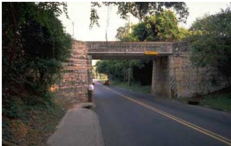
All facilities should end logically, with a reasonable warning, and an alternative route, so that the user is not suddenly “trapped.”
