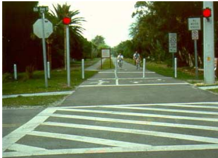
This trail provides sufficient warning for both motorists and bicyclists of the approaching mid-block crossing. There is also a push-button signal to ensure that they can cross safely.
