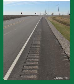
Edge rumble strips are milled corrugations in pavement to alert inattentive drivers that they are leaving the roadway to reduce:
