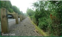
Roadside and median barriers are designed to redirect and slow vehicles while shielding them from obstacles likely to result in a more severe crash, such as:
