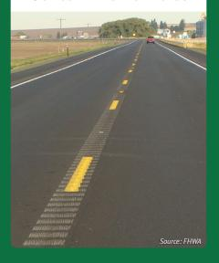
Center rumble strips are milled corrugations in pavement to alert inattentive drivers that they are crossing the center line to reduce:
