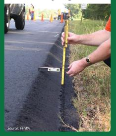
SafetyEdge<sup>SM</sup> is a paving technique producing a durable 30-degree edge to prevent tire-scrubbing, which often results in:
