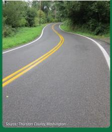
Retroreflective pavement markings improve nighttime highway visibility. Wider lines (6"–8") have an increased safety effect, reducing:
