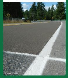
HFST is a pavement surface treatment using calcined bauxite that provides exceptional skid-resistant properties at high friction demand locations such as curves, ramps, or intersections where problems with wet conditions, speed, or geometrics contribute to:
