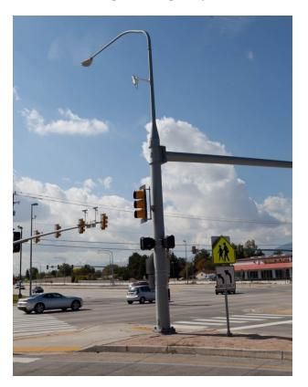
Exhibit 1-10. Lighting, pedestrian signage, and video detection at the right-turn channelization at the Bangerter Highway/3500 South Intersection in Utah.<sup>(2)</sup>
