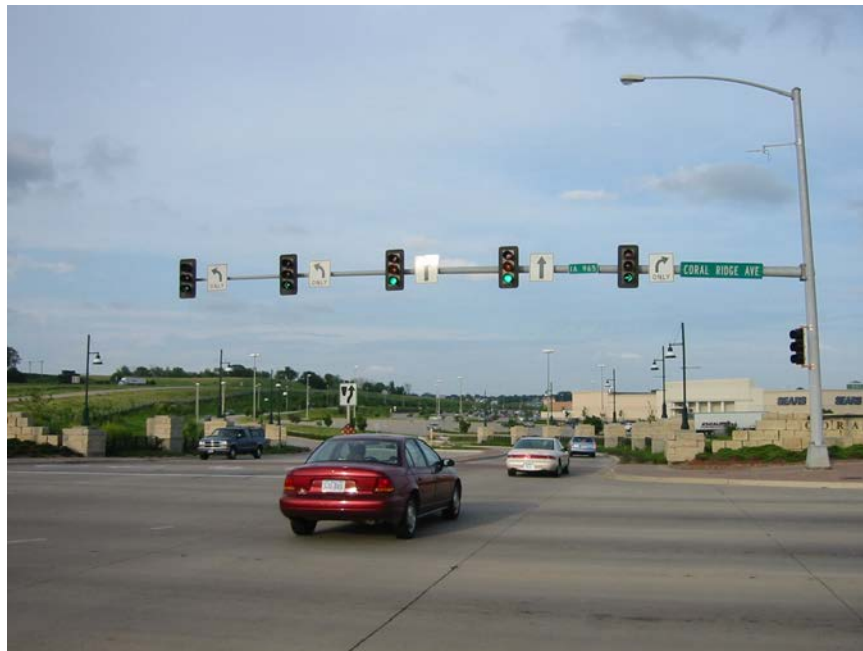
Exhibit 10-7. Lane-aligned signal heads.
