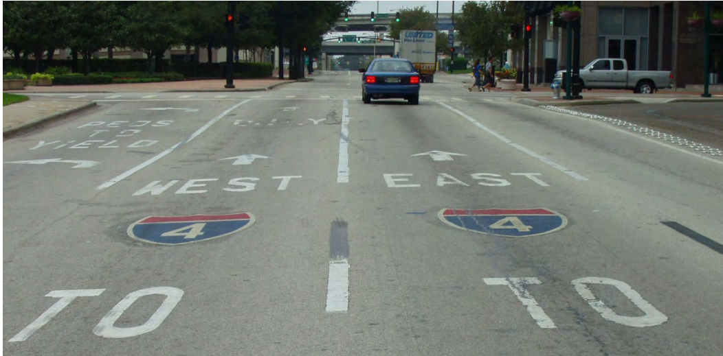
Exhibit 5-23. Example of pavement legends indicating destination route numbers (“horizontal signage”).
