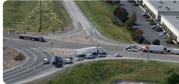
Trucks Using a DDI in Salt Lake County, UT Source: DDI Video FHWA-SA-14-019
