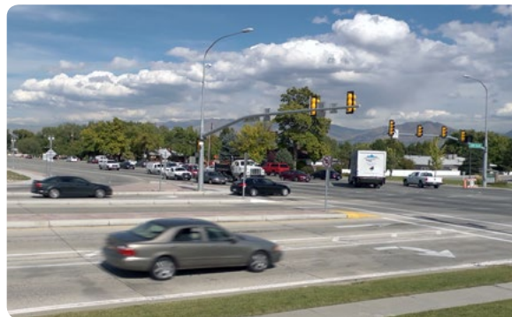
DLT Intersection at 6200 South and Redwood Road Source: DLT Case Study Video FHWA-SA-14-057
