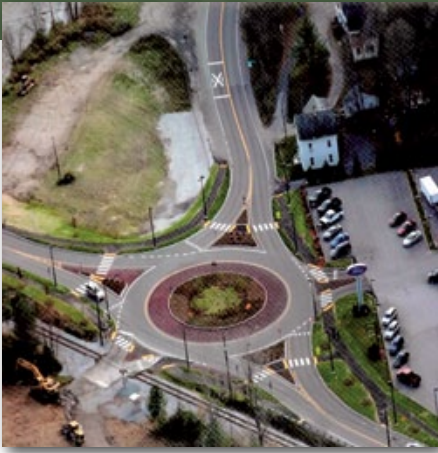
Figure 1: Overhead photo of the second roundabout completed in Montpelier.
