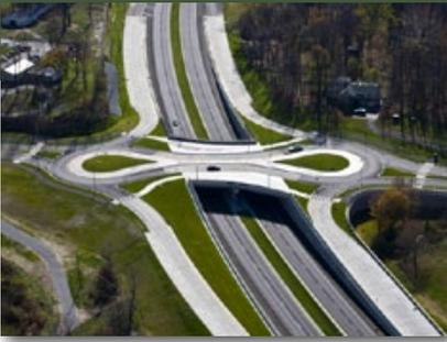
**Figure 2:** Overhead photo of the completed roundabout installed above the Keystone Parkway at 136th Street.
