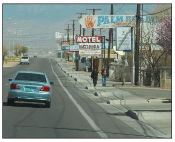
Exhibit 14: A corridor with closely spaced driveways creates a challenging environment for pedestrians and bicyclists. Pedestrians with mobility restrictions may be particularly affected by driveways through sidewalks. These locations require careful design and construction to ensure they meet requirements under the American with Disabilities Act (ADA). (Source: VHB)
