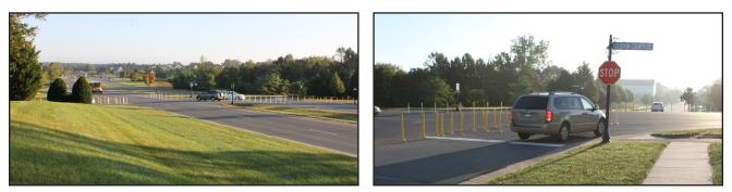
Exhibit 2: At this location, corridor access management measures were implemented to reduce crashes at median crossovers. Flexible post-mounted delineators were installed to restrict direct left turns from the side street. The photo on the left shows the main street and two vehicles in the median turning left onto the side street. The photo on the right shows how the delineators were placed to prevent vehicles from turning left through the median onto the main street. (Source: VHB)
