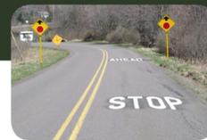
**I2 – Provide a double yellow centerline on the median opening of a divided highway at intersections**
