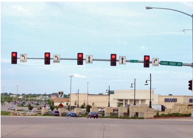
Figure 3: Example Intersection with Basic 12 inch Lens, Back Plates and a Signal Head per Lane
