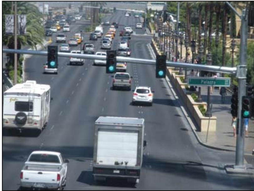
**Figure 3: Example of backplates on a multilane arterial intersection**
