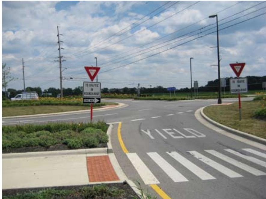
**Figure 4: Example of entry to multi-lane roundabout**
