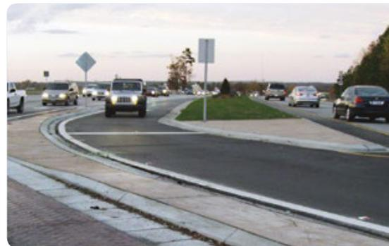
Vehicle Turning at an RCUT Intersection Along the NC 55 Bypass
