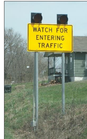
Advance intersection warning sign. Source: MoDOT.
