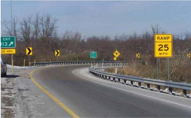
***Installing chevron signs on horizontal curves can produce a 16 percent reduction in non-intersection fatal and injury crashes.***
