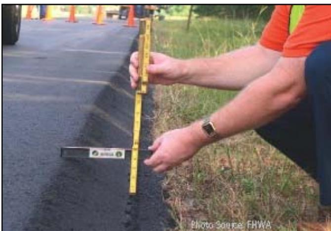
**The benefit-cost ratio of using Safety Edge<sub>SM</sub> on two-lane roads is very high, ranging from 4 to 63.**
