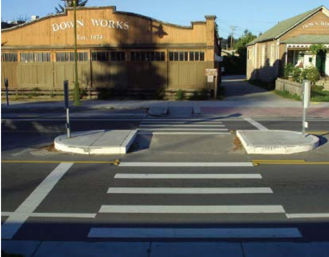
Example of a pedestrian refuge island. Source: www.pedbikeimages.org/Dan Burden
