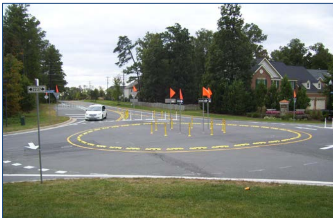
The “instant roundabout” at the intersection of Poland Road and Edgewater Street in Loudoun County, Virginia reduced crashes by 89 percent. Image courtesy of VDOT.
