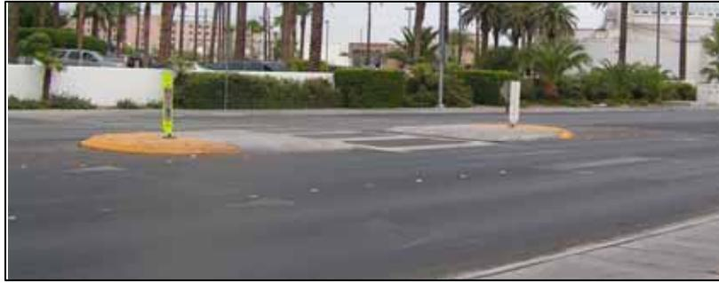
**Figure 37. Median Refuge Island at Mid-block Location in Las Vegas**
