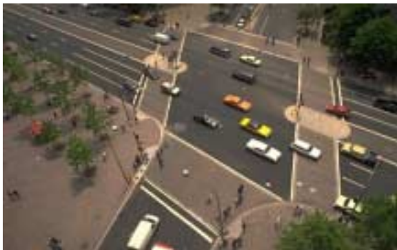
Use of colored crosswalks and median refuges makes this intersection more pedestrian-friendly.
