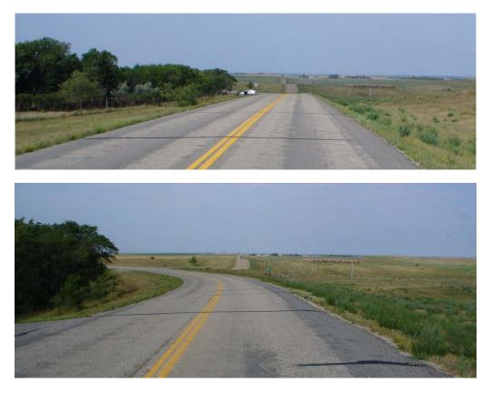
Figure 62. Photo. An example of a visual trap exists when a crest vertical curve blocks the view of the upcoming horizontal curve (top photo). What appears to be a continuation of the road in the distance is actually an intersecting roadway in the midst of a curve (bottom photo).
