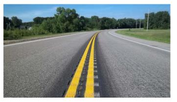
Figure 5. Photo. Centerline rumble strips.
