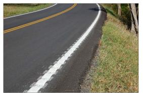
Figure 48. Photo. Milled Edge Line Rumble Stripes. Source: KYTC.
