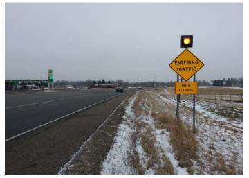
Figure 65. Photo. A dynamic warning sign alerts drivers in real time of other users in the roadway.
