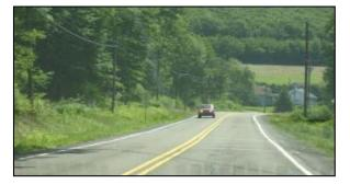
Figure 10. Photo. Roadway with 4-inch edge line.
