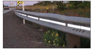
Several States have experimented with using retroreflective paint, tapes or panels in the web of the W-beam.
