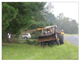
Figure 50. Photo. Removing brush as part of clear zone maintenance. Source: Texas DOT.
