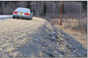
Figure 51. Photo. Typical barnroof slope design. Source: Alaska DOT.
