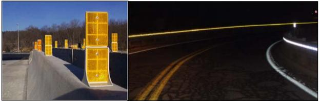
Figure 57. Photo. Delineated concrete Fig barriers. Source: Michigan DOT.
