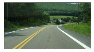
Figure 11. Photo. Roadway with 8-inch edge line.
