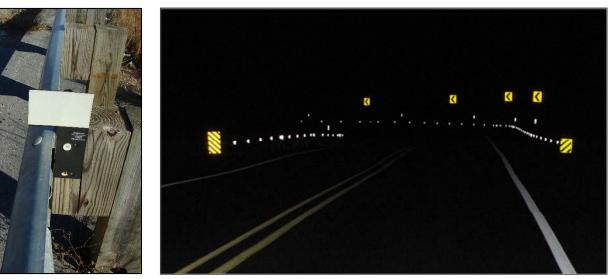
Figure 56. Photo. Delineators installed on post, nighttime view. Source: Michigan DOT.
