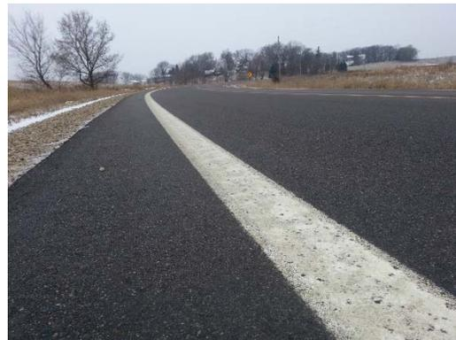
**Figure 7. Photo. Delineation with enhanced (6-inch) edge lines.**
