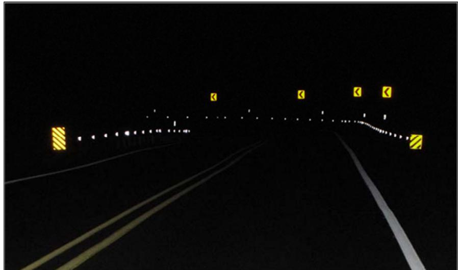
**Figure 56. Photo. Delineators installed on post, nighttime view. Source: Michigan DOT.**
