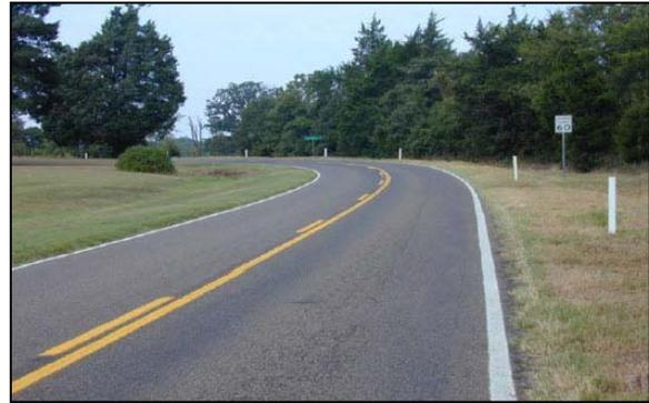
**Figure 12. Photo. The color of delineators must match the color of the adjacent edge line.**
