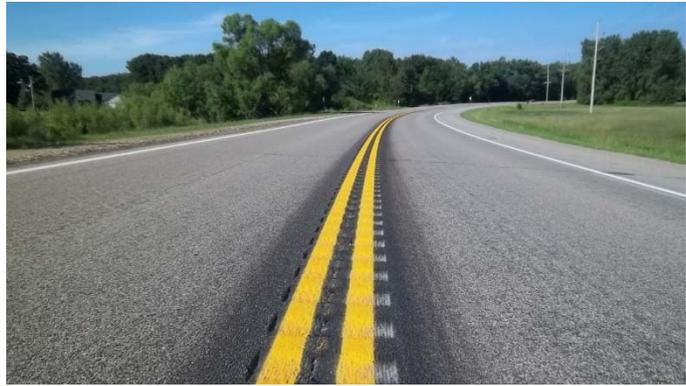
**Figure 5. Photo. Centerline rumble strips.**
