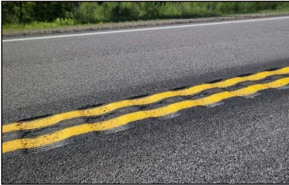
**Figure 47. Photo. Milled Center Line Rumble Stripes.**
