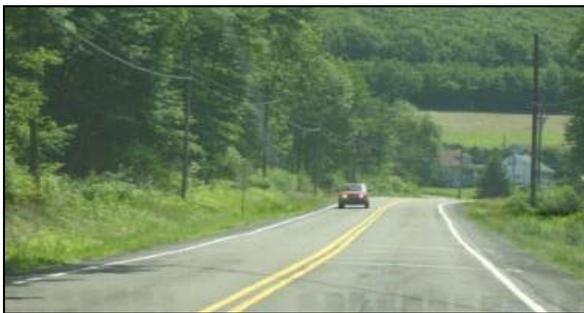
**Figure 10. Photo. Roadway with 4-inch edge line.**
