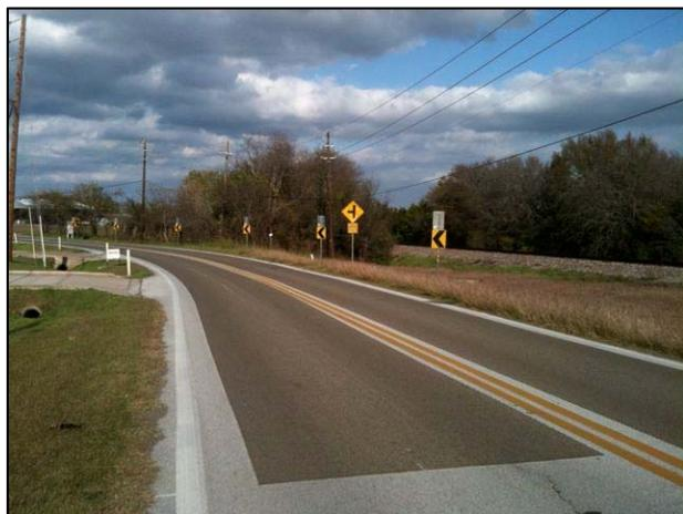
Figure 41. Photo. HFST on a horizontal curve.
