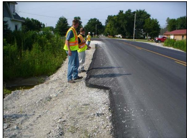
**Figure 44. Photo. Shoulder paving operation.**
