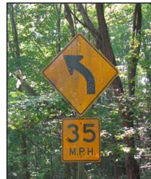
Figure 38. Photo. Low Retroreflectivity sign example.
