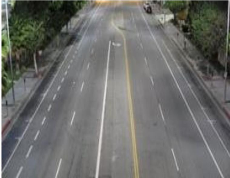
*The lighting along this roadway provides relatively uniform illumination well within the recommendations of IES RP-8.*
