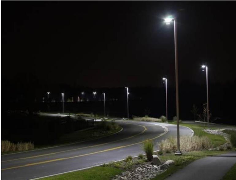
*Continuous lighting along a curve on an access road at night provides good illumination along the roadway.*
