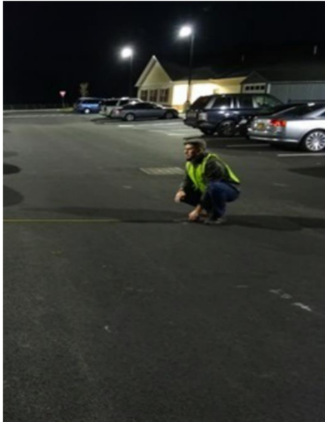
A worker laying out a grid to take lighting measurements.
