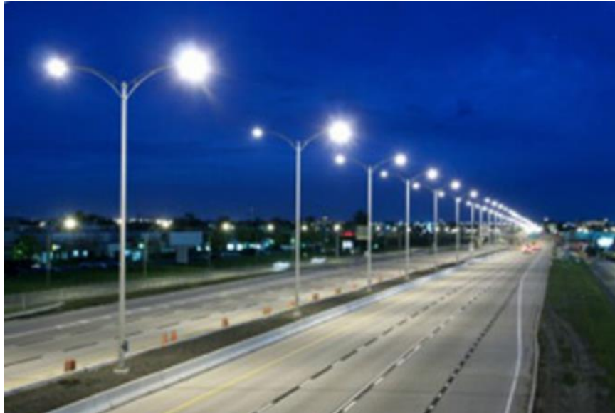
An expressway with relatively uniform lighting.
