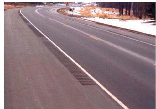
Gapped shoulder rumble strips allow bicycle flow between shoulder and driving lane.
