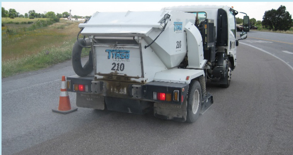
Figure 19. Photograph. Example of aggregate removal using a power broom.
