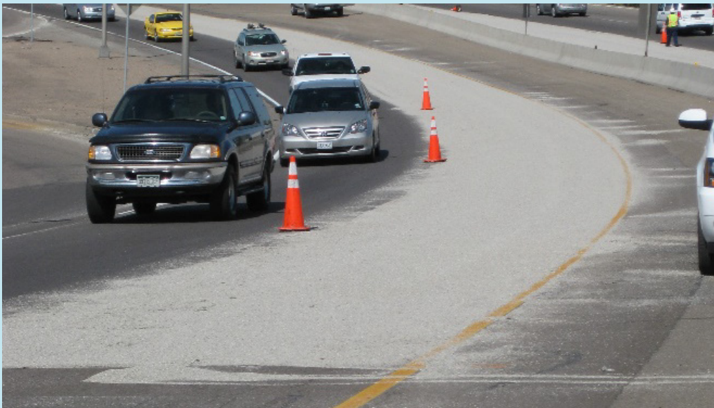
Figure 21. Photograph. Example of exposure of underlying pavement after sweeping.
