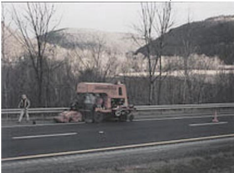
**FIGURE 2. New York State's Milled Rumble Strip Design**
