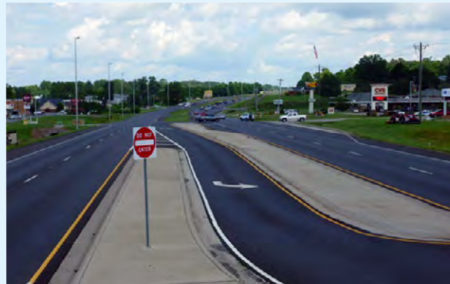
An off-set left turn lane provides additional site distance and decreases the number of sideswipe-type crashes.
