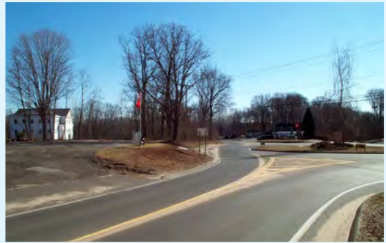
Before: Rotary prior to conversion. Note lack of deflection from entrance on far side of the photo.
