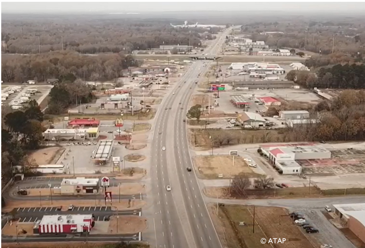
Figure 2. Photo. Aerial photo of the prior condition of W South Boulevard between I-65 and Davenport Drive.
