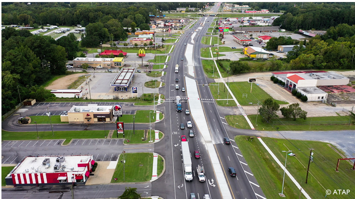
Figure 5. Photo. Aerial photo of completed W South Boulevard improvements.
