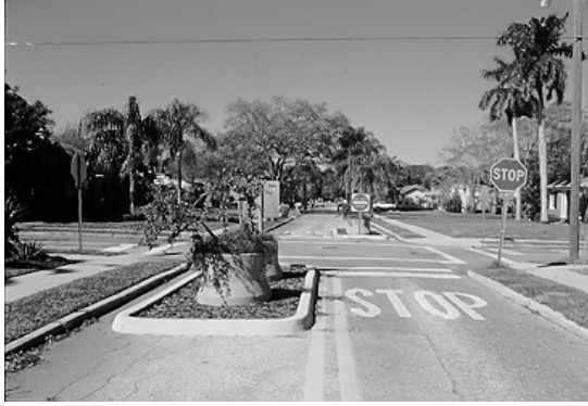
Figure 5.19. Semi-Diverter. (Irving St.—Sarasota, FL)
