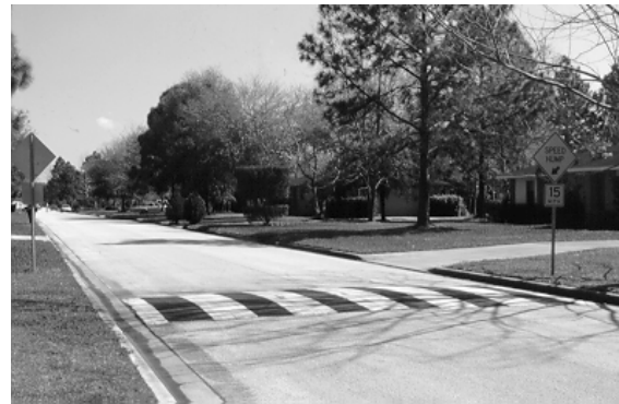
Figure 6.2. New Tool in Toolbox—12-foot Speed Hump. (Gainesville, FL)
