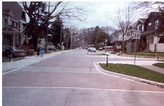
Raised Intersection with Neckdown. (Toronto, ON, Canada)
