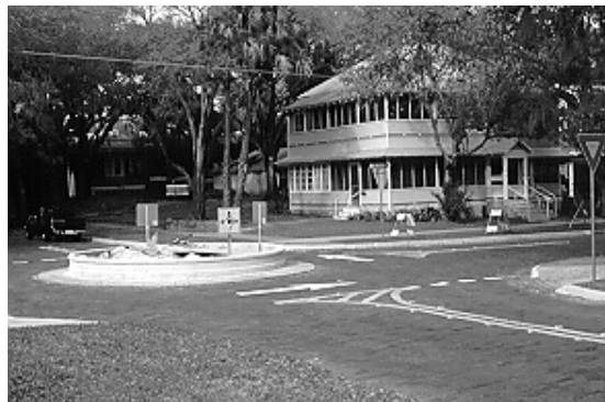
Figure 7.13. Traffic Circle with a 2-inch Lip to Accommodate Fire Trucks. (Orlando, FL)
