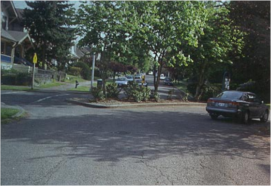
Truncated Diagonal Diverter. (Seattle, WA)
