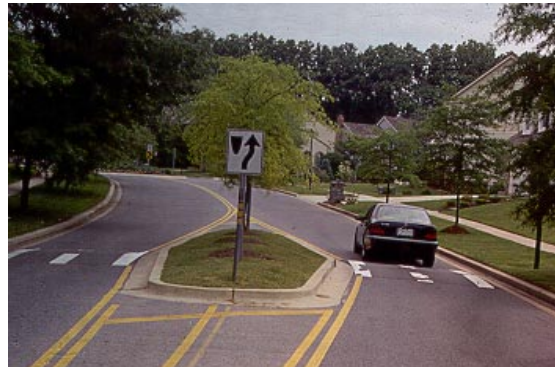
Center Island with Humps. (Montgomery County, MD)
