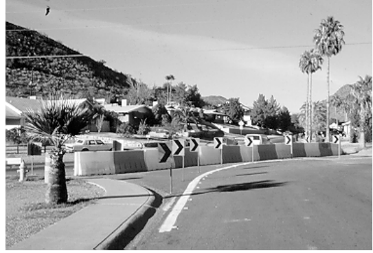
Figure 5.16. Diagonal Diverter. (6th Ave.—Phoenix, AZ)
