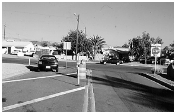
Figure 7.11. Half Closure that Invites Violations. (Phoenix, AZ)
