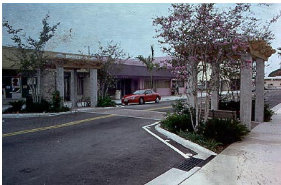
Raised Crosswalk with Choker. (West Palm Beach, FL)
