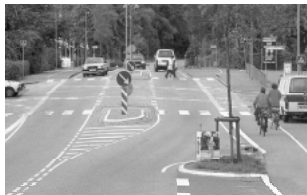
Figure 9.4. Reallocation of Right-of-Way with Deflection.
