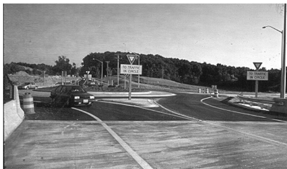
Figure 9.19. High-Capacity Interchange Roundabout. (Howard County, MD)
