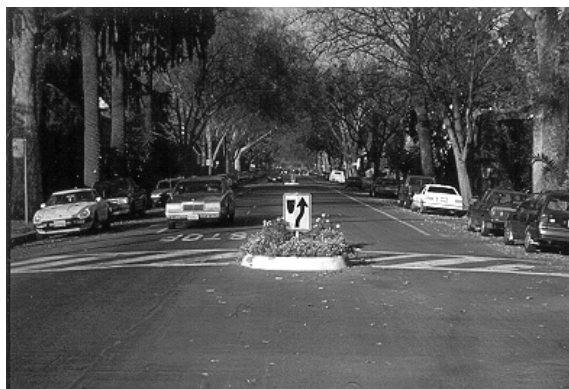
Figure 9.21. Commuter Route Converted Back to Two-Way Operation—and Traffic Calmed at the Same Time. (Sacramento, CA)
