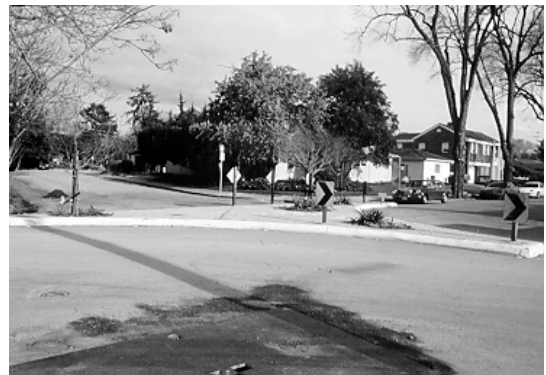
Figure 5.18. Diverter/Closure. (17th St.—San Jose, CA)
