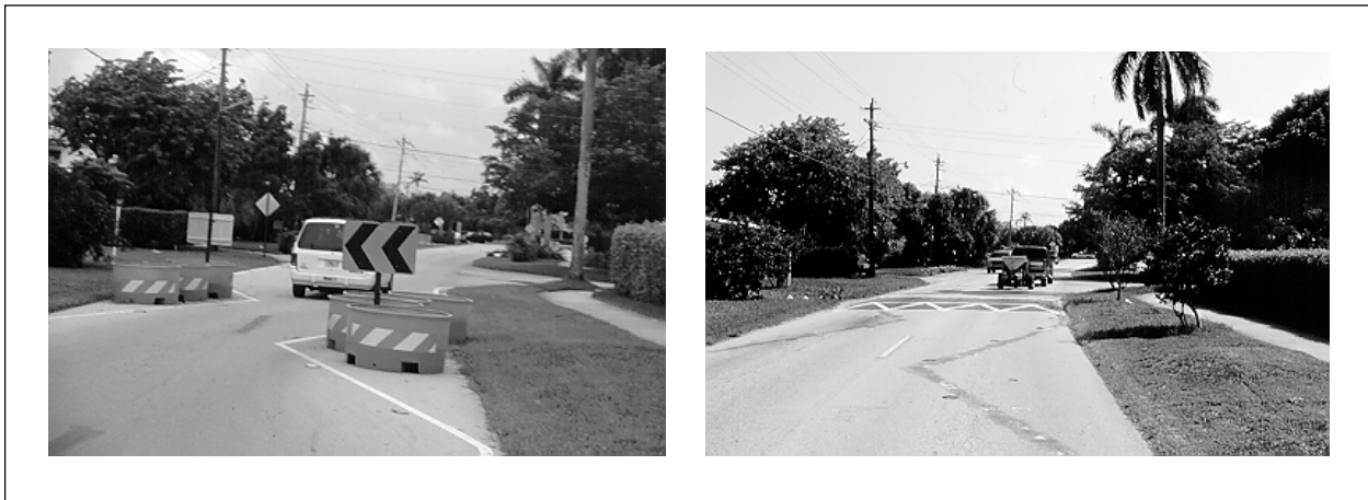
Figure 9.15. Temporary One-Lane Choker and Speed Table that Replaced it. (Ft. Lauderdale, FL)
