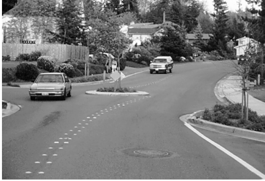
Figure 5.13. 18-foot Diameter Traffic Circle with Neckdowns. (SE 46th Way—Bellevue, WA)
