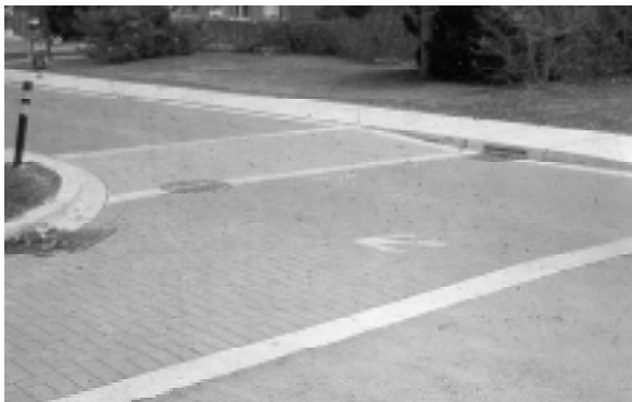
Figure 7.26. Gradual Ramp on a Raised Intersection. (Toronto, ON)
