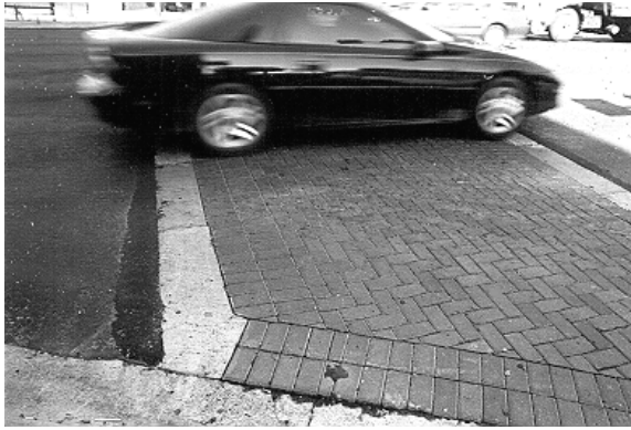
Figure 9.16. Crosswalk Reconstructed to Be Less Bump-Like. (Tallahassee, FL)
