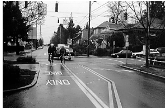
Figure 7.12. Half Closure that Discourages Violations. (Portland, OR)
