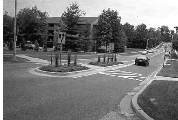
Figure 3.33. Center Island Narrowing with a Break for a Crosswalk. (Montgomery County, MD)
