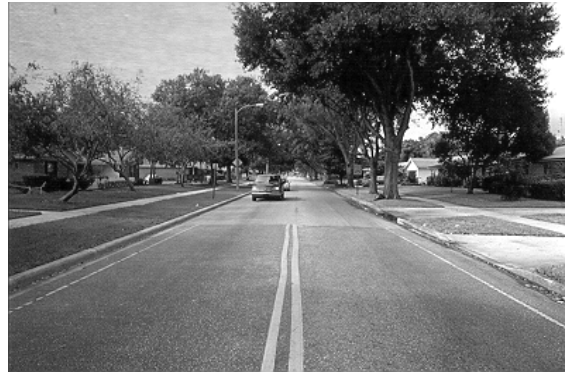
Figure 5.47. Remnant of Visual Narrowing that Proved Ineffective. (Orlando, FL)
