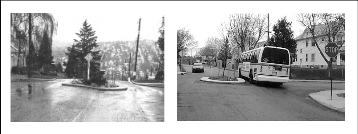
Figure 3.19. Traffic Circles with Cutouts for Transit Vehicles. (Seattle, WA, and Dayton, OH)
