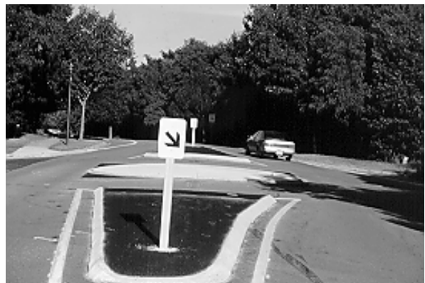
Figure 4.22. Concrete-Topped Circle Controversial for Its Aesthetics. (Howard County, MD)
