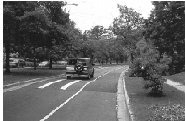
Figure 6.9. One of More than 1,100 Speed Humps in Montgomery County, MD.
