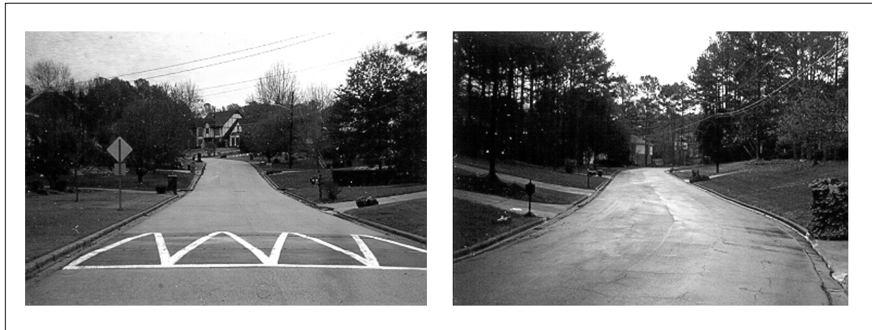
Figure 5.36. Two Phases of the Same Development— One Traffic Calmed and the Other Not. (Gwinnett County, GA)
