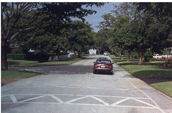
22-foot Hump. (Ft. Lauderdale, FL)
