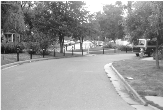
Figure 7.15. Diagonal Diverter with Removable Bollards. (Boulder, CO)
