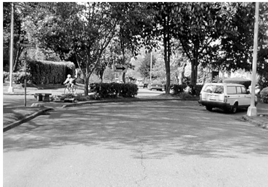
Figure 5.20. Diagonal Diverter. (16th Ave. E.—Seattle, WA)
