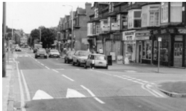
Figure 2.4. Raised Intersection in a 20-mph Zone. (Manchester, England)
