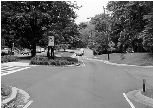
Figure 5.14. Chicanes/22-foot Speed Tables. (Huntington Pkwy.—Montgomery County, MD)
