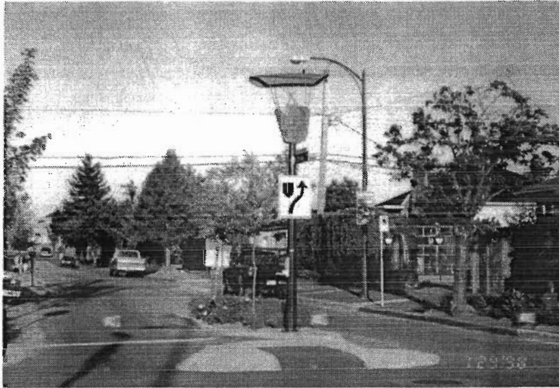
Figure 3-10. Central Island Narrowing with Landscaping and Artwork in Vancouver, CAN.
