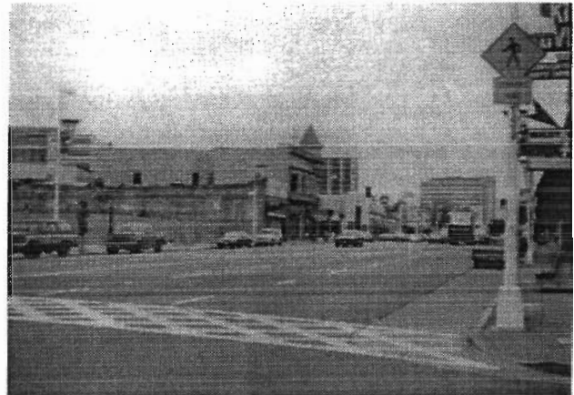
Figure 4-10. Lattice Crosswalk Markings in Oakland, CA.
