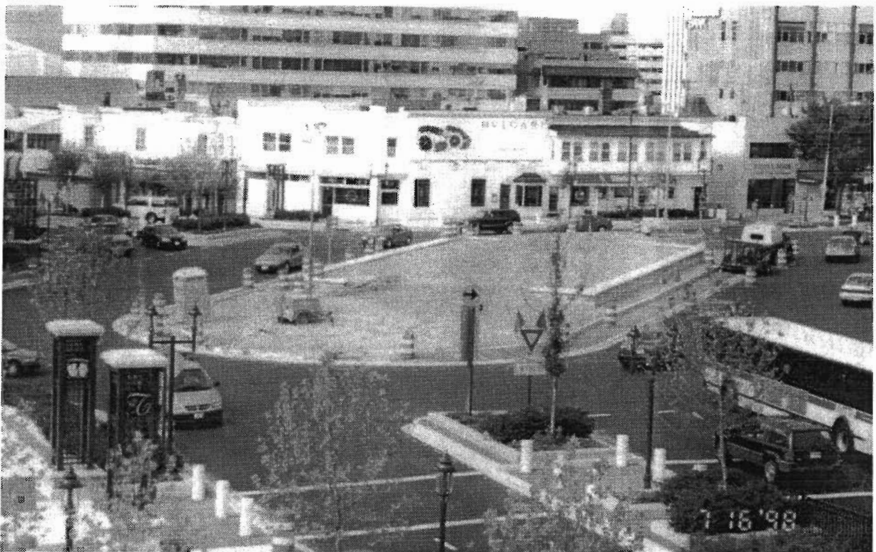
Figure 3-53. Oval Roundabout Under Construction in Towson, MD.
