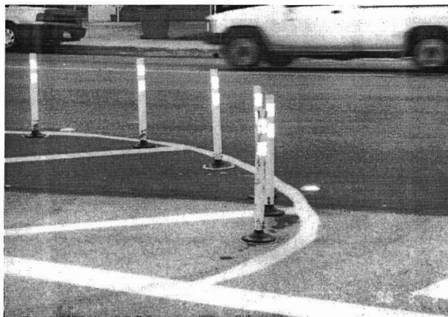
Figure 3-28. Semi-diverter in Glendale, CA.
