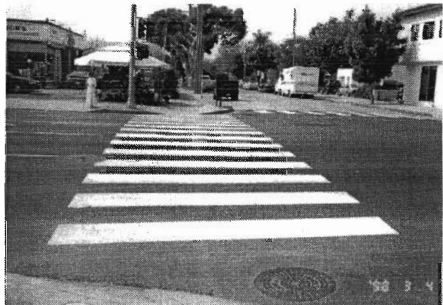
Figure 4-12. Ladder Style High-Visibility Crosswalk in Santa Barbara, CA.
