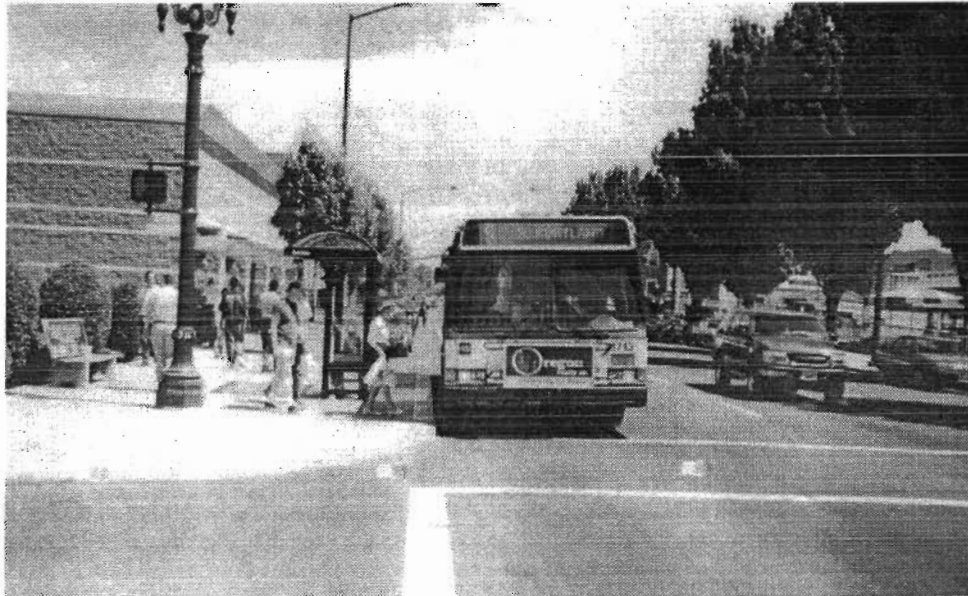
Figure 3-6. Bus Stop at a Neckdown (also known as a Bus Bulb) in Seattle, WA.
