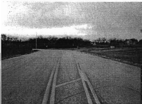
Figure 3-14. Painted Median to Indicate Roadway Narrowing.
