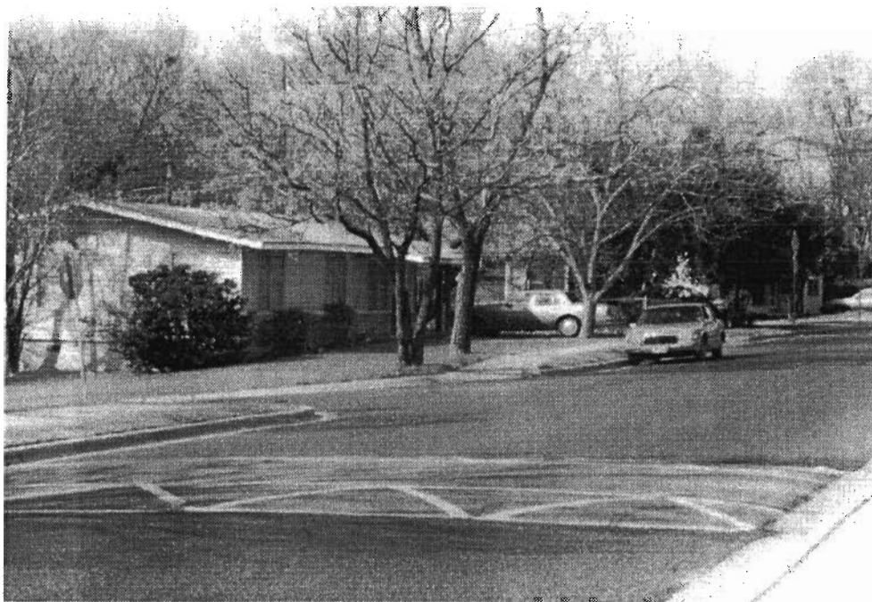
Figure 2-1. Speed Hump in Austin, TX.
