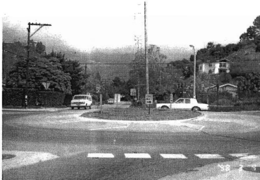
Figure 3-47. Roundabout in Santa Barbara, CA.
