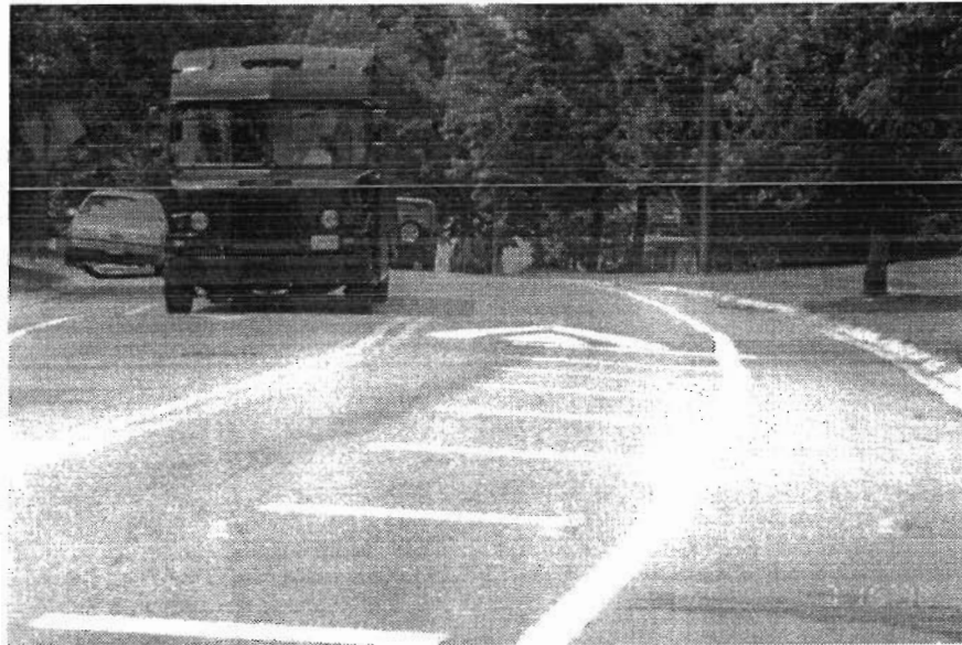
Figure 4-30. Transverse Pavement Markings in Montgomery County, MD.
