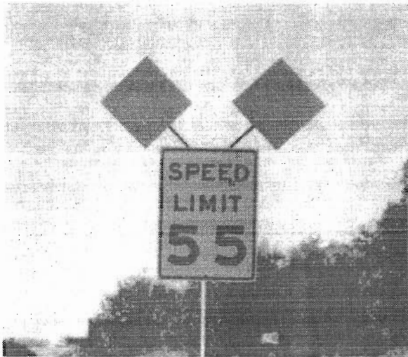
Figure 5-18. Orange Metal Flags on Speed Limit Signs in Rochelle, TX.
