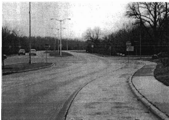
Figure 5-11. Multi-way Stop Signs in Garland, TX.
