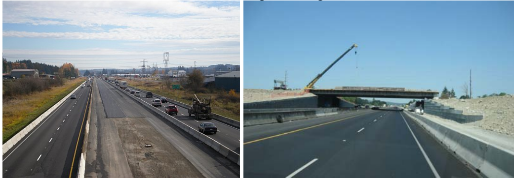
Figure 3: I-5 Rush Road construction zone changes during automated enforcement.
