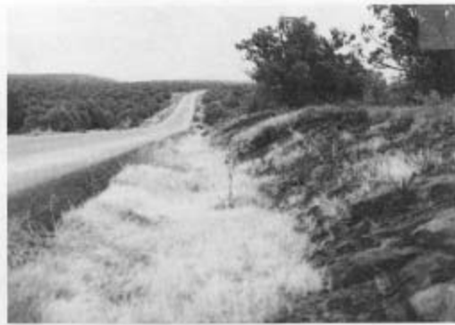
Rural roadside hazard rating of 3.
