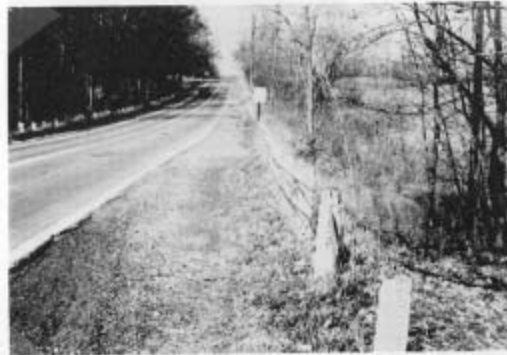
Rural roadside hazard rating of 5.
