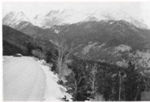
Rural roadside hazard rating of 7.
