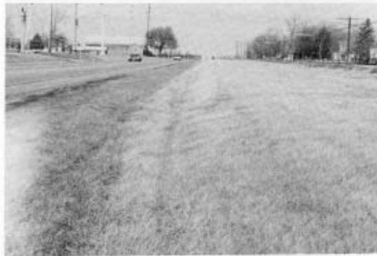
Rural roadside hazard rating of 1.
