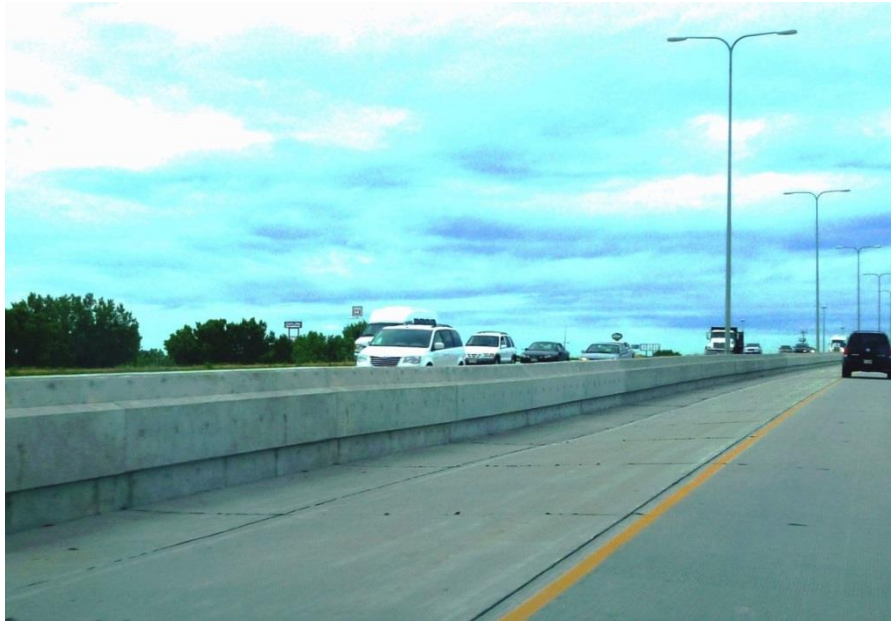
Figure 5. Photo. TL-5 concrete median barrier.
