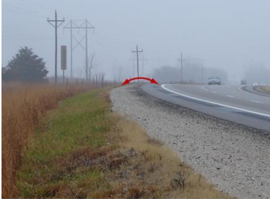
Figure 4. Photo with illustration. Cross-slope break on a superelevated curve.
