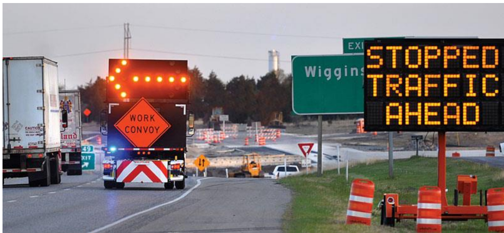
Figure 21. Photo. Dynamic queue detection warning sign in a work zone.
