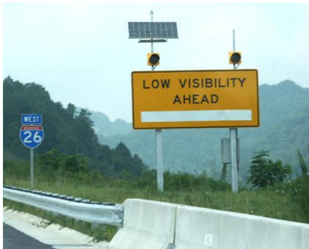
Figure 22. Photo. Weather advisory system using a static sign with beacons.
