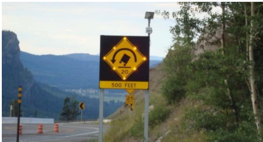
Figure 17. Photo. Dynamic warning sign showing activated truck rollover warning system.
